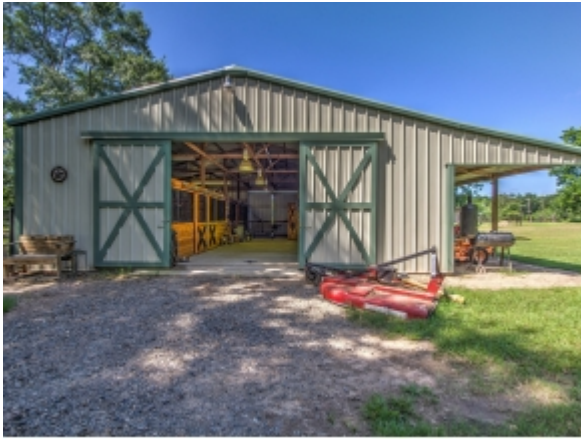
The Metal Barn
