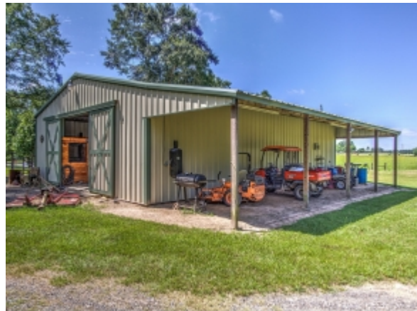
Side of Metal Barn
