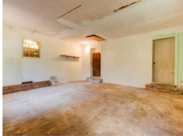
Unfinished Garage enclosed
